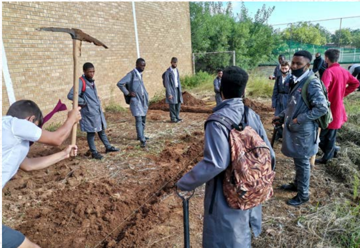
Learners construct the steel frame of the hen house
