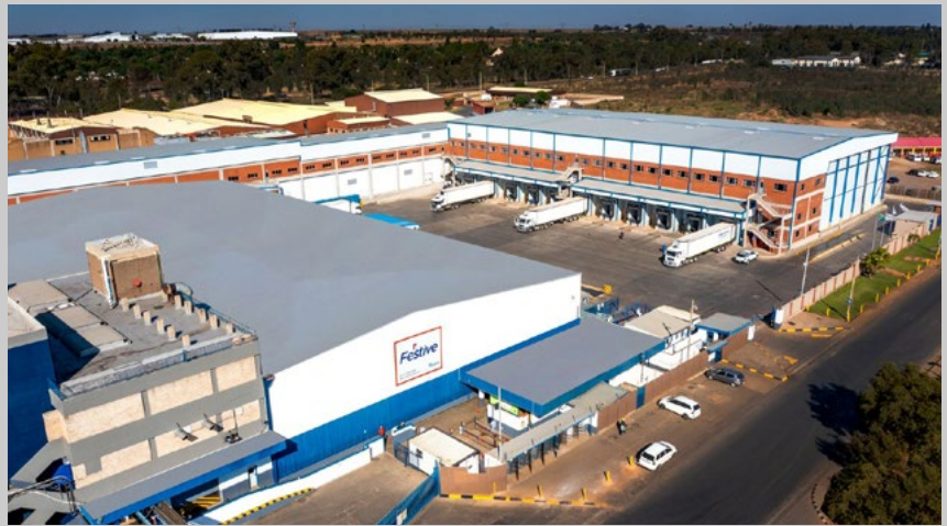
Astral's investments have delivered some of the most technologically advanced facilities in South Africa, such as the Meadow Feeds feed mill in Standerton and the Festive processing plant in Olifantsfontein (below)
