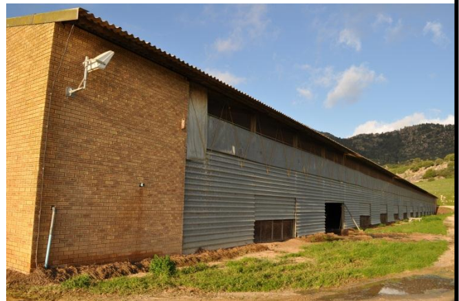
High rise building for layers in cages on the right, note openings for removal of manure from side-openings
