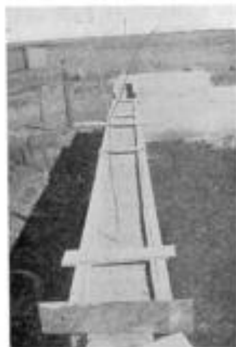
Fig. 1.—The mould filled with the mixture. Note projecting wire to be attached to the beams.
